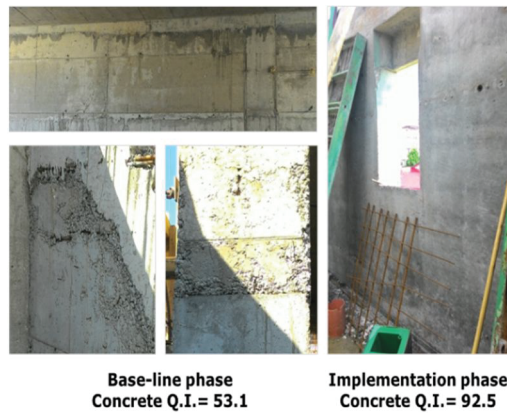
Fig. 8 – Comparison of the quality of concrete works between the two phases of the study
