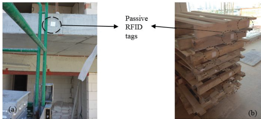
Figure 4: Passive RFID tags on (a) building floors, and (b) masonry block pallets
