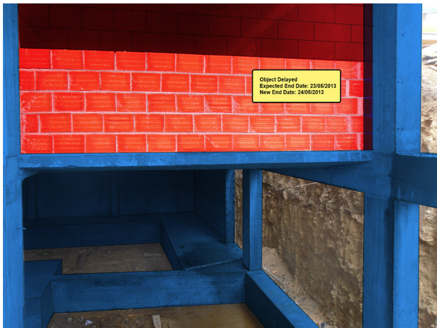
Fig. 5: Example of a tag note assigned to a delayed wall with relevant information
