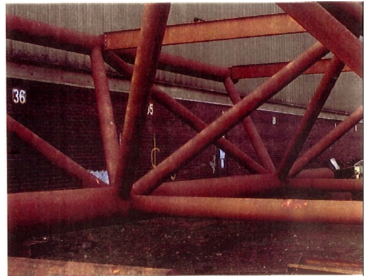
Figure 4. Part of the manufactured sub-assembly (Cleveland Bridge UK Ltd)
