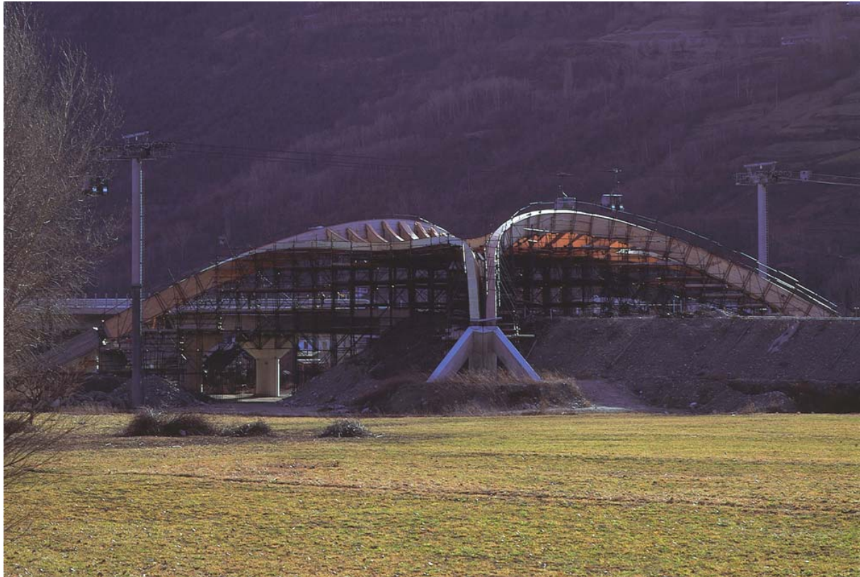
Figure 11. The structure completed with the temporary scaffolding still up.
