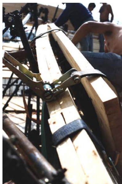
Figure 10. Stacking process of a timber leaf.
