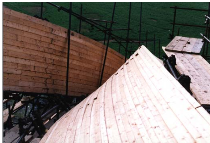
Figure 7. Two beams converging toward the bearing.
