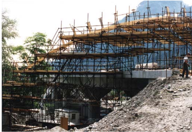
Figure 9. Temporary scaffolding with the templates and the first layers of timber.
