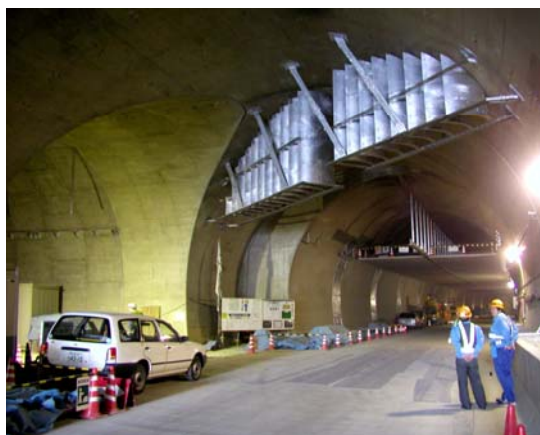
(a) Whole View of Corner Vane Fixed Situation
