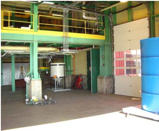
Figure 1. Existing facility structure
