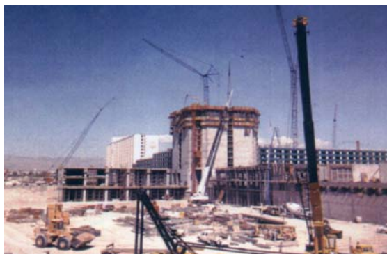
Figure 1: MGM Grand Hotel Construction Site
