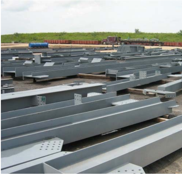
Figure 3. Grid storage of steel components
