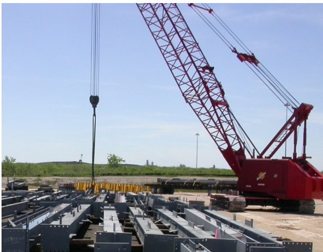
Figure 1. Crawler-mounted lattice crane lifting a heavy column
