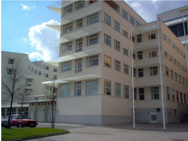
Figure 2: The fifth wing project at Jönköping University: a prefabricated concrete building containing offices and lecture halls.
