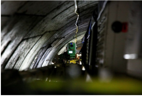
Figure 3. Robotic total station.
