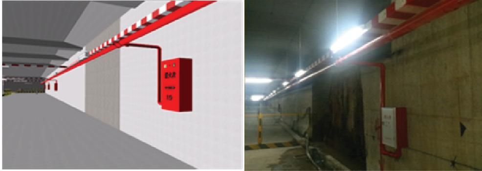
**Figure 8** A screenshot of the 3D model related to an order sheet for the installation of a fire box and a photo on site after the work was completed
