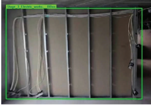
Figure 2: Stage 3-Electrical and plumbing works
