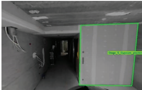
Figure 3: Stage 6: Plastering of the wall
