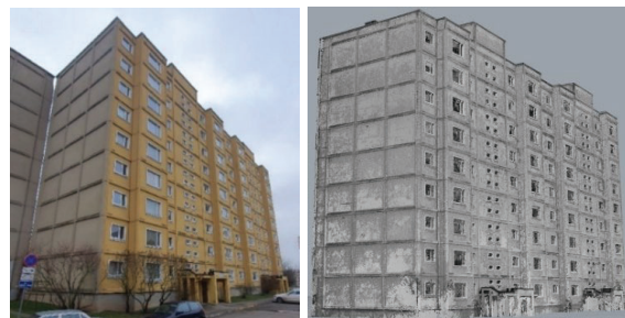
Figure 1: A typical apartment building in Estonia (picture on the left and point cloud on the right) that need to be renovated by using industrialised and digitalised renovation processes
